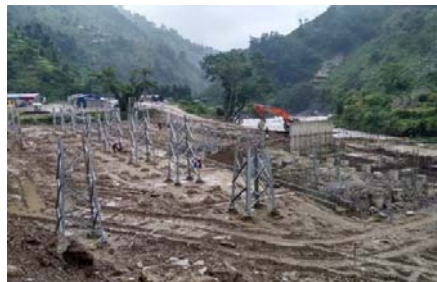
Erection in progress at Likhu A switchyard
