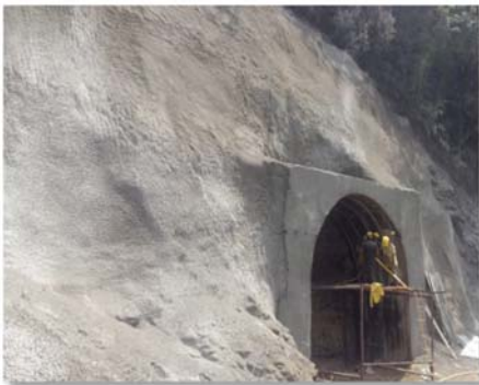
Portal under construction
