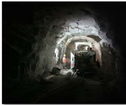
Drilling in progress for Tunnel construction
