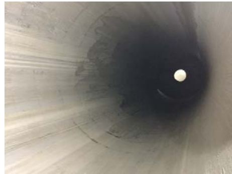
Vertical Shaft after concrete lining
