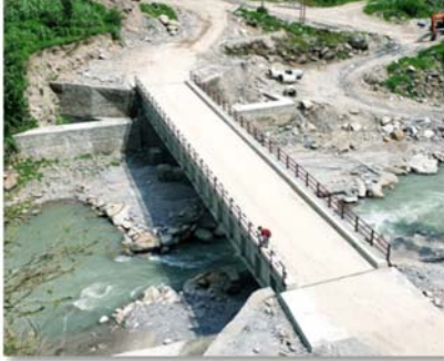
35 meter span plate Girder Bridge at Kinja
