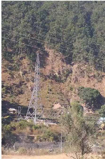
End Point Transmission Tower Erection Completed
