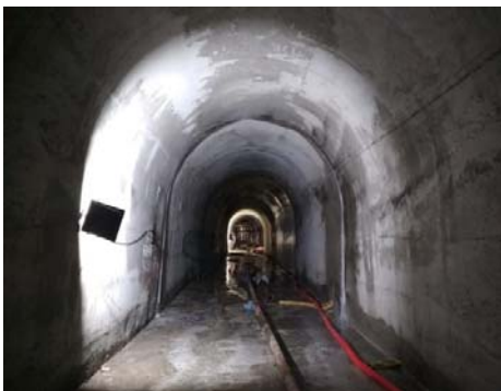
Tunnel after Concrete Lining
