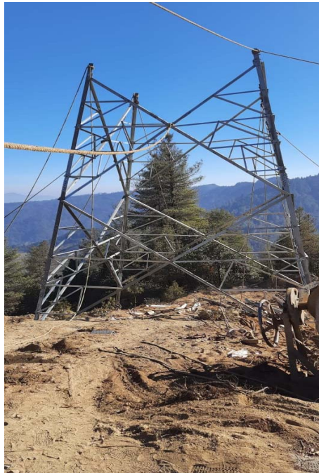
Angle Point Tower Erection in Progress
