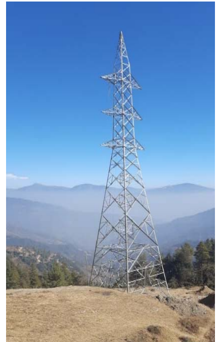
Angle Point Tower Erection Completed
