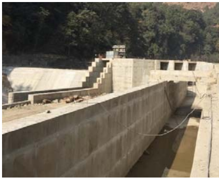
Headworks of Likhu 'A' Hydropower Project
