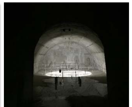
Tunnel after Invert Lining
