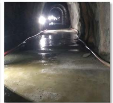
Tunnel after Invert Lining
