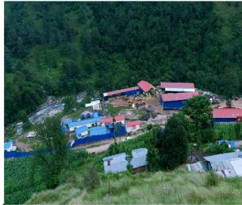
Industrial Shed constructed for a construction site
