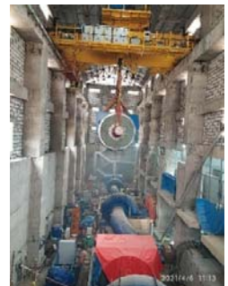
Power House Building
