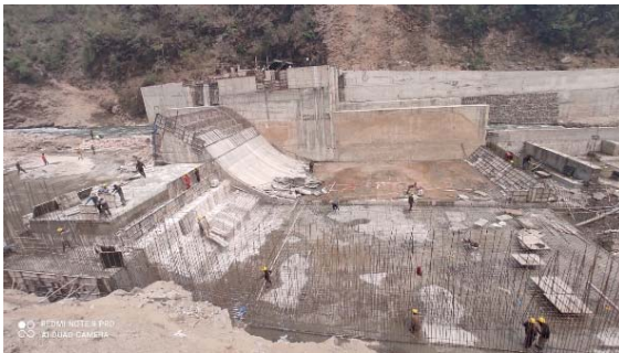
Weir under Construction for at Likhu 2 HEP
