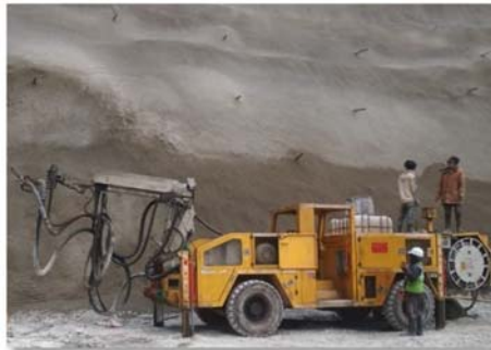
Shotcreting in Progress for Slope Stabilization
