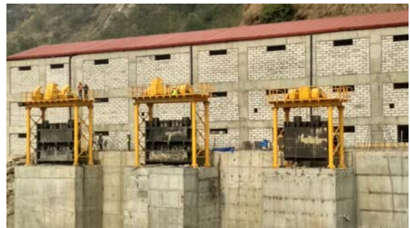
Power House Building
