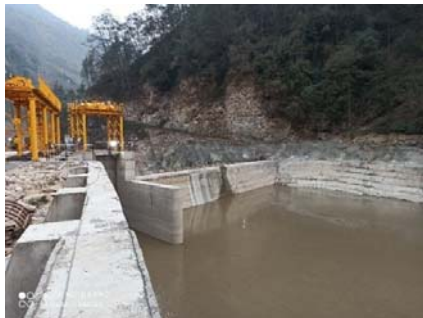
Likhu A Headworks after Completion
